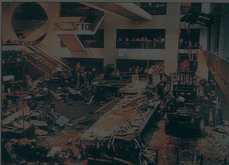
Lobby of the Hyatt Regency Hotel in Kansas City after the walkways collapsed
